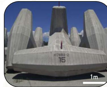
Wave-dissipating blocks with uneven surface
